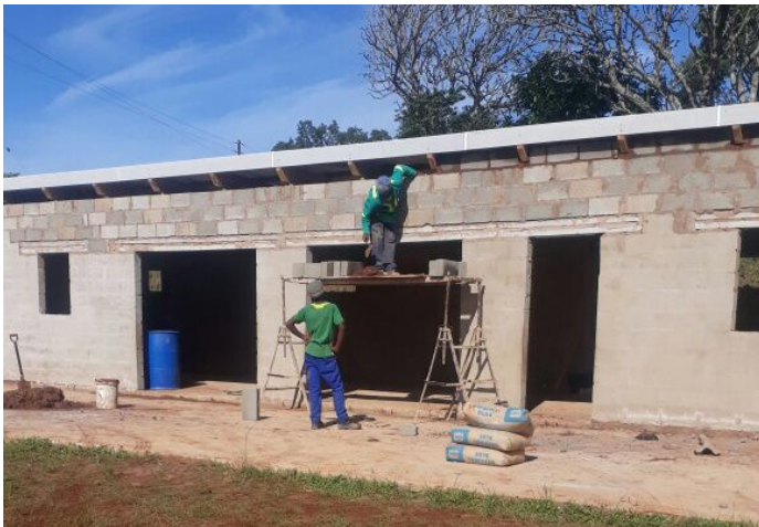
Construction of the new building
