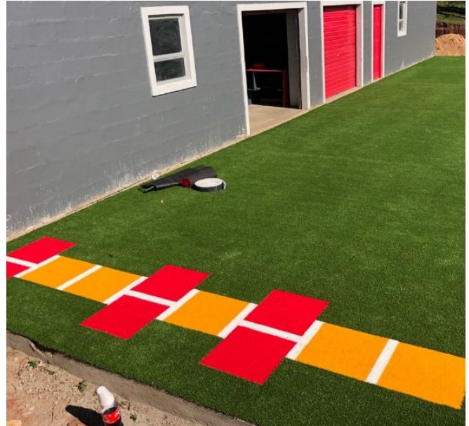
Donated Astro Turf installed on the Verandah
